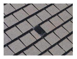
Replace damaged shingles.
