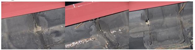
Remove old sealant, clean, apply compatible roofing cement/sealant.
